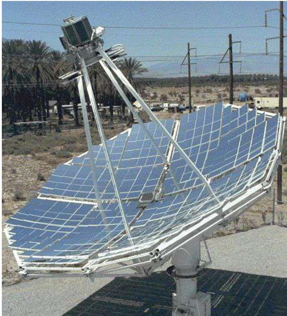
**Advanco/Vanguard 25 kW dish /Stirling system installed at Rancho Mirage, California.**
