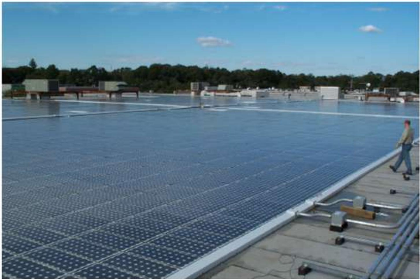
Crystalline silicon array in flat roof mounting
